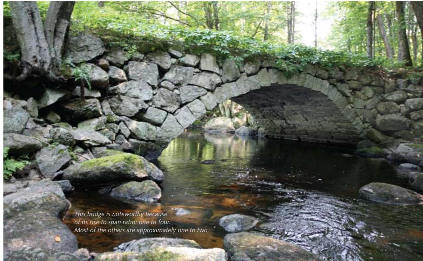
This bridge is noteworthy because of its rise to span ratio: one to four. Most of the others are approximately one to two.
