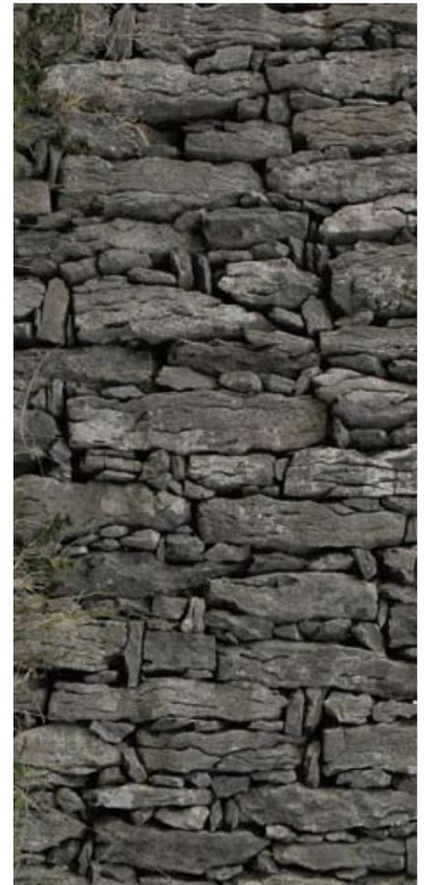
A properly built vertically coursed wall is similar to a horizontally coursed wall with respect to the primary rule of stonemasonry: "one over two, two over one"—*except* that in a vertically coursed wall it should be one *against* two, and two *against* one. The photo above is a section from the wall in the photo to its left. It has been rotated 90 degrees. Note how much this looks like a well-built horizontally coursed wall.
