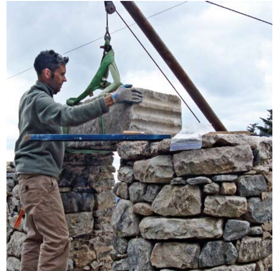
Using the gin-pole to set the lintels.
